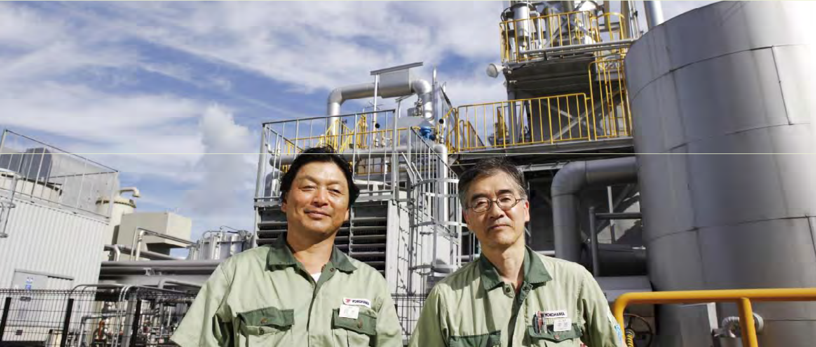
General Manager Toshihiko Suzuki (left) and Deputy General Manager Kenji Teraoka in front of the cogeneration system at the Shinshiro Plant, which boasts a total efficiency of at least 85%
