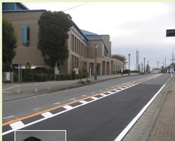
Masato Kokusho and a section of road in front of the Zama City Office in Kanagawa surfaced with the porous elastic road-surfacing material for testing (November 2006)
